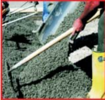
Figure 4: Placing of PAVESCAPE Concrete
