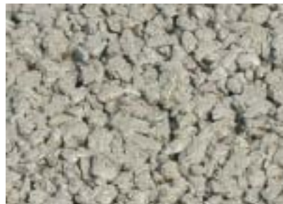
Figure 2: Closer View of PAVESCAPE concrete
