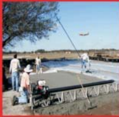
Figure 5: Compaction of PAVESCAPE Concrete
